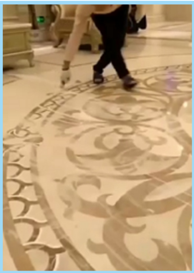
Scraping: Poma repair powder and fine tapping 3H
